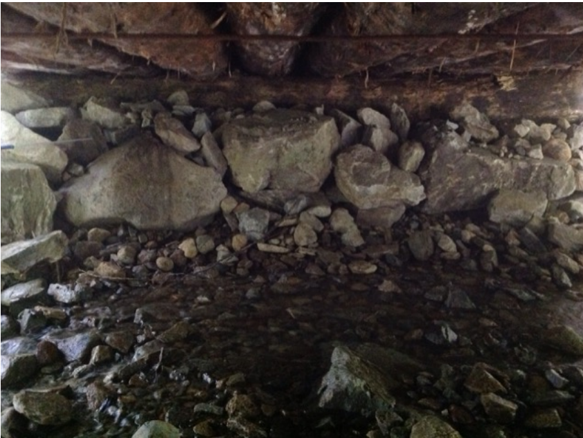
Right Bank Abutment when facing downstream
