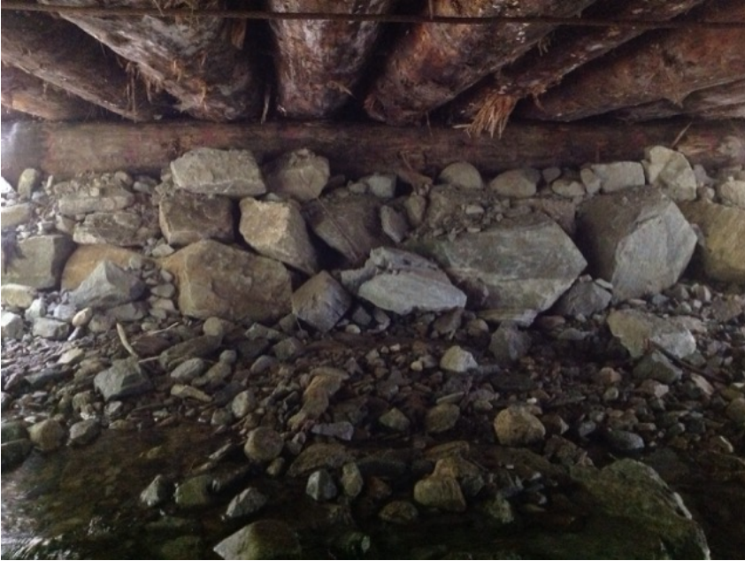
Left Bank Abutment when facing downstream
